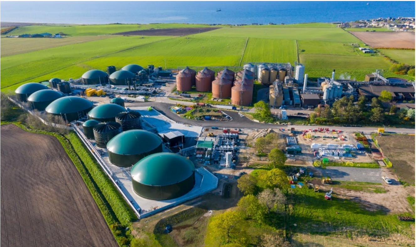
Figure 4: Biomethane facility connected to our network in Scotland
