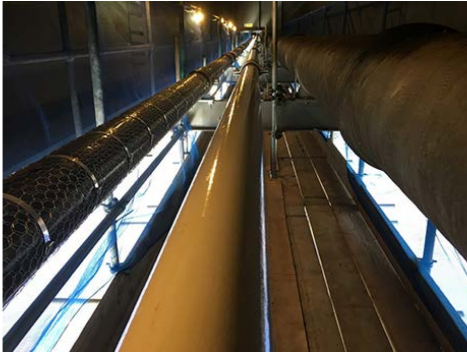
A view alongside the pedestrian bridge. We're replacing the old 12" steel gas main with a smaller six inch steel pipe (centre)
