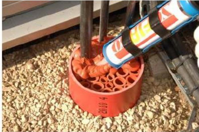
Figure 3.5: Sealing of a service duct
