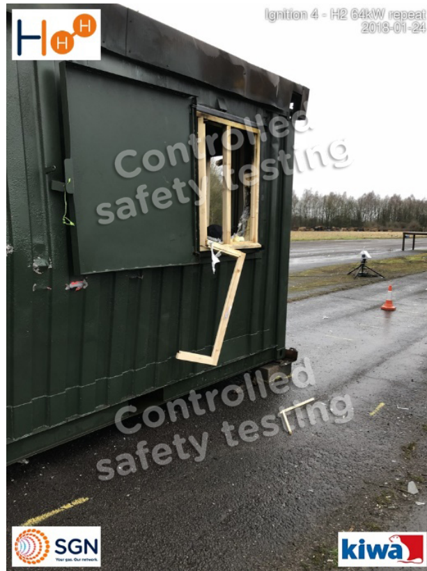
Figure 46: Outside view of damage to FIB shape on opposite side to sink cupboard, also showing blown out window
