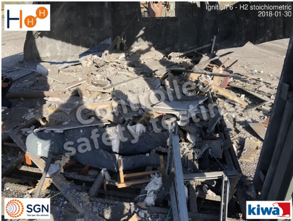
Figure 56: Close up of damage inside FIB showing collapsed ceiling, walls and floor, and 30kg dummy and broken chairs
