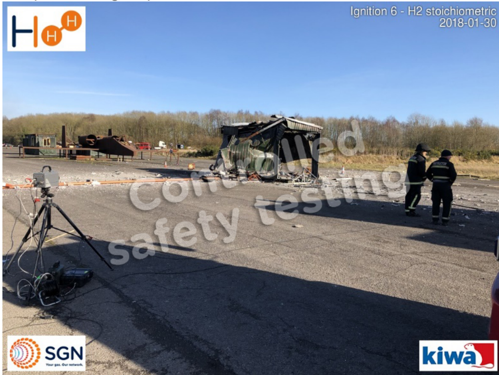
Figure 54: Wide view of severely damaged FIB and extent of debris on runway (approx. 25m in both directions)
