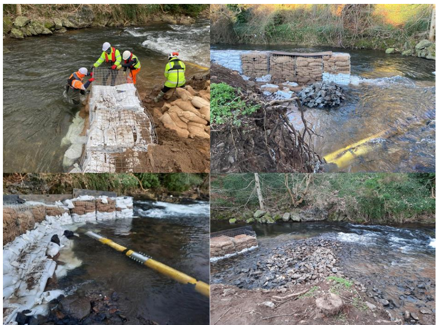
Figure 5: Stages of rock dumping to remediate washout.
