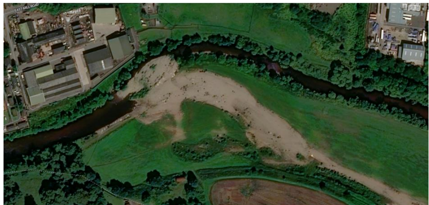
Schematic 2 – River South Esk at Brechin in 2024. Satellite imagery shows the impact of Storm Babet at the be where the riverbank protection (and foliage) has been washed away.
