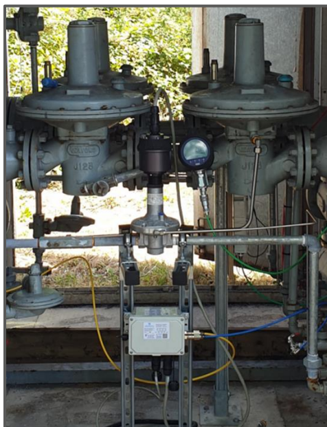
Figure 5: Remote Pressure Management Actuator and Control System
