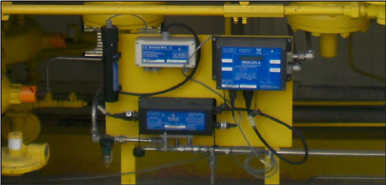
Figure 2 details a typical gas profiler and logger system.
