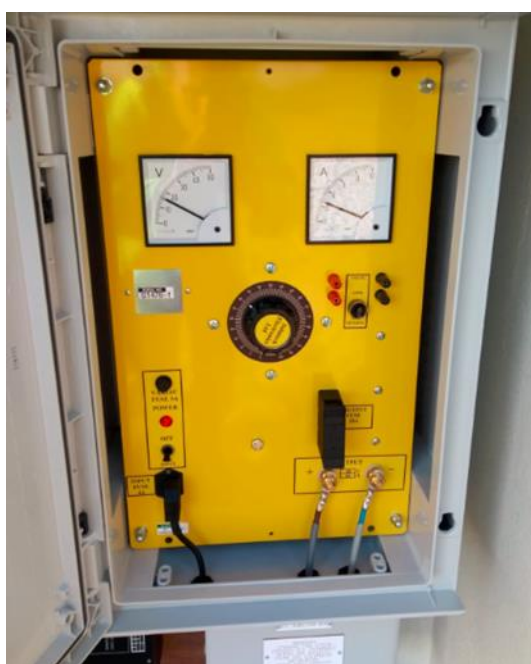
Figure 5: Newly installed TR
