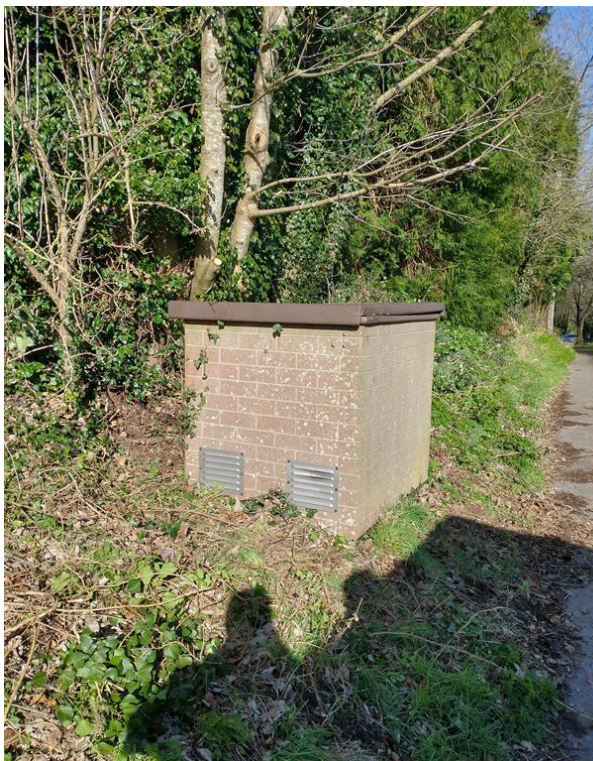
Figure 2: Housing Replacement at Tidworth Road, Hampshire
