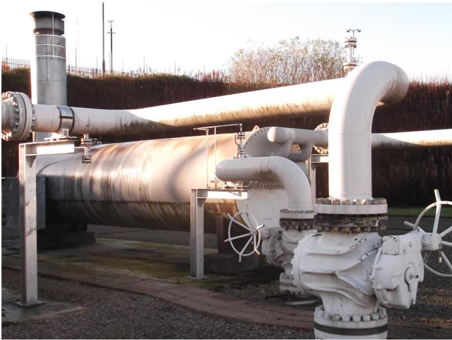
Figure 2: Shell and Tube Heat Exchangers Hardwick Offtake
