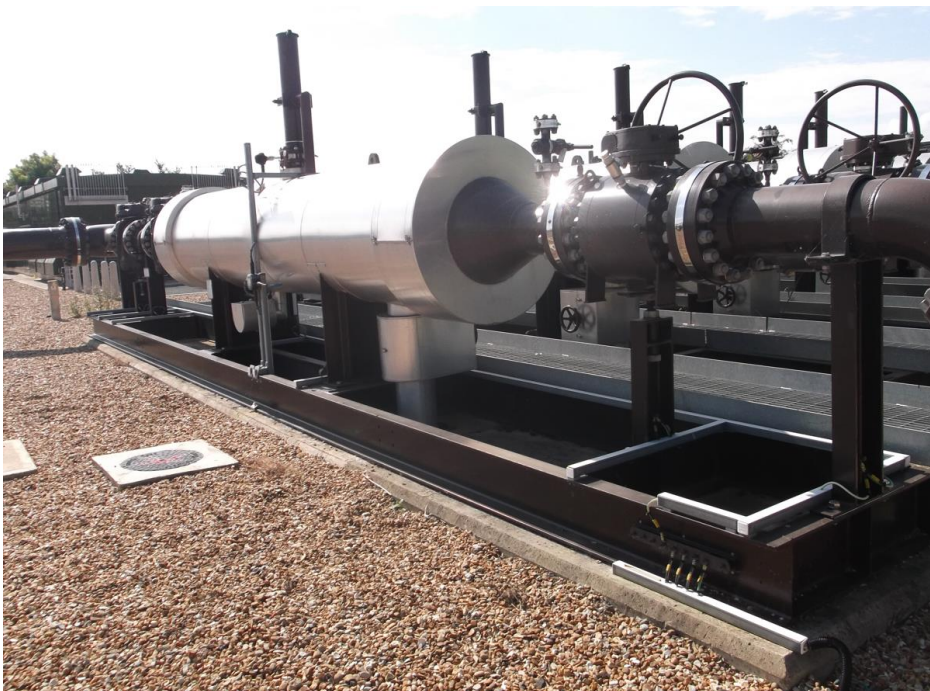
Figure 2: Shell and Tube Heat Exchangers Hardwick Offtake
