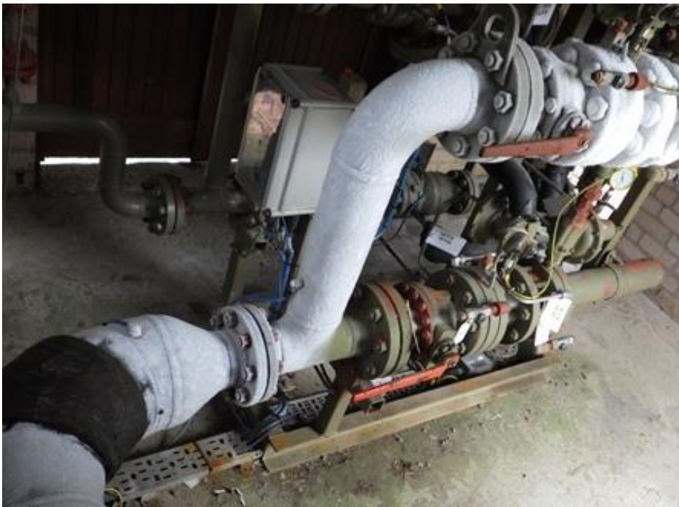
Figure 10: Example of the effect on outlet pipework on a site without pre-heating
