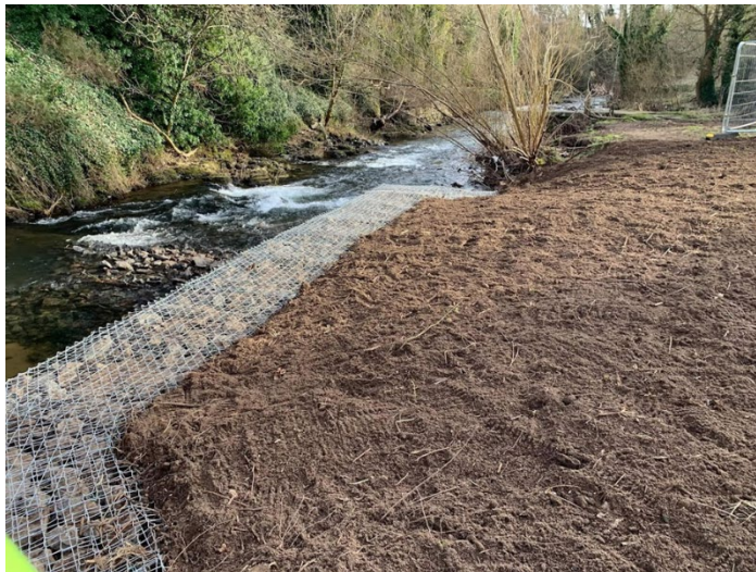
Figure 8: Reinforcement of riverbank.
