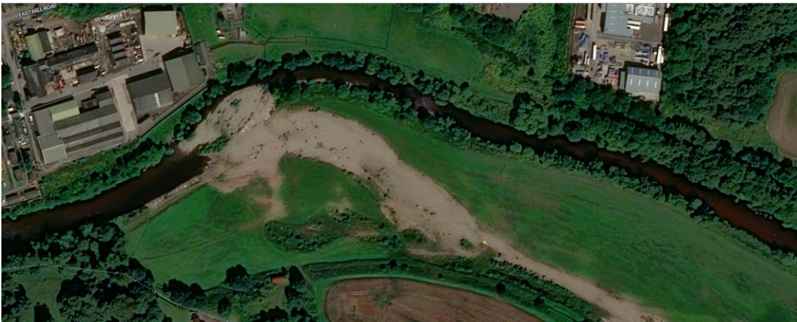
Schematic 2 – River South Esk at Brechin in 2024. Satellite imagery shows the impact of Storm Babet at the bend of the river where the riverbank protection (and foliage) has been washed away.
