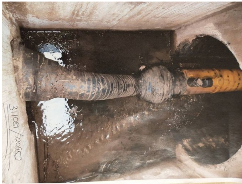
Figure 2: Gas culvert prior to Storm Babet, free flowing and free of debris
