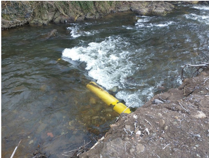
Figure 6: Exposed section of IP pipe crossing River Dighty
