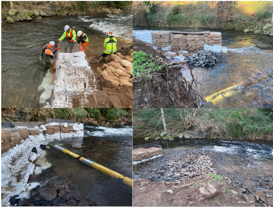
Figure 7: Stages of rock dumping to remediate washout.
